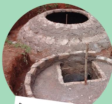
Biogas digester installed at a smallholder dairy farm
