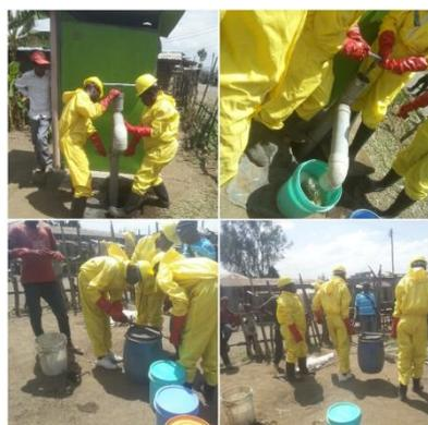
Working closely with the Public Health Office and County Government, NCSP developed an innovative safe and hygienic emptying and transport of faecal sludge suitable for LIAs. The Gulper technology has been tested, pit-emptier associations are engaged and a Primary
