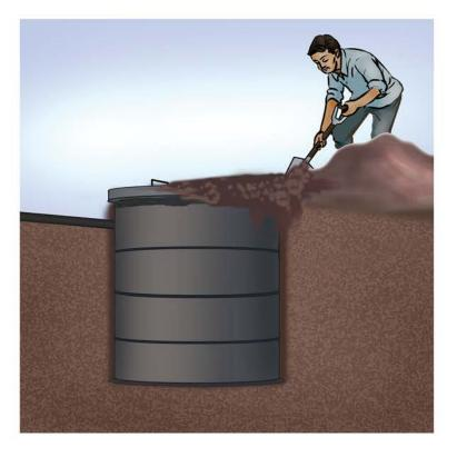
• Pit should be covered by soil to minimum above the handles of RCC slab for safety purpose
