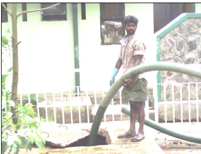
Figure 2: Emptying Operation of FS from a Septic Tank Using Vacuum Equipment
