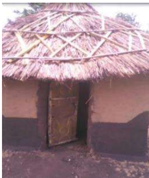
Complete pit latrine. Image: Uganda Country Team
