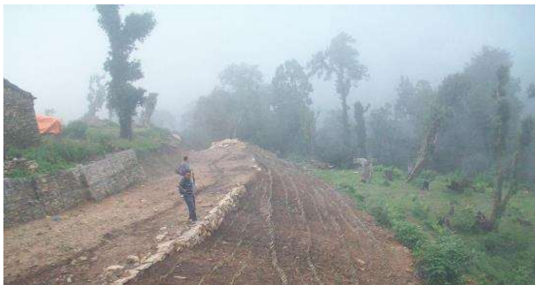
Bio-engineering plantation to prevent landslides at Dungeshawor RM, Dailekh, Nepal. Image: Ram Singh
