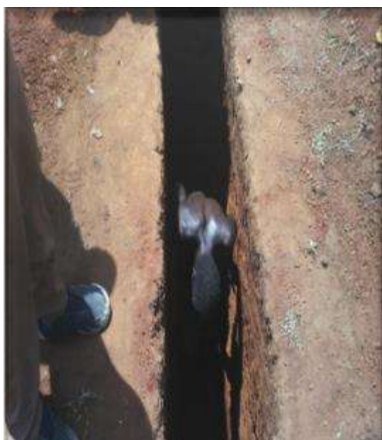
Excavation of pit latrine. Image: Uganda Country Team
