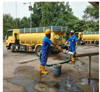
Mechanical sludge emptying in progress. Photo credit: SNV Indonesia and Rajeev Munankami/WASH SDG project supported by DGIS.
