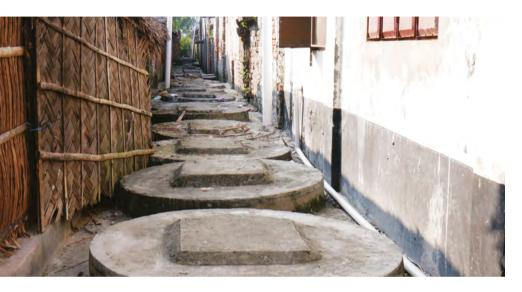
household, and maintenance is limited to regular emptying of the settler, and cleaning of the filter.
