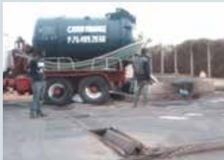
Damaged liquid recovering drain
