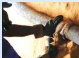
pipes connected with plastic bags and inner tube
