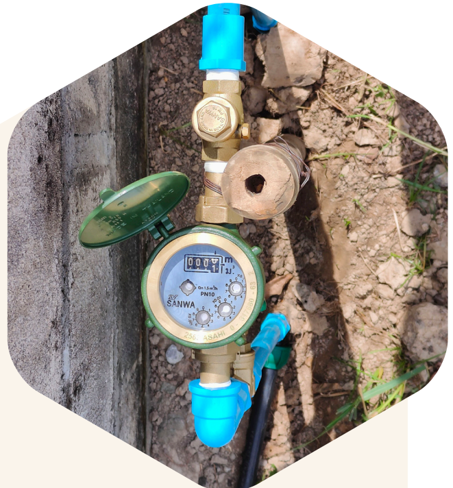
Photo: A household water metre connection to the state-owned water provider utility in peri-urban Champhone District.
