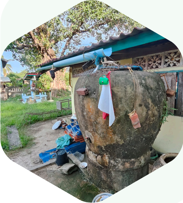
Photo: A large rainwater jar and collection system.
