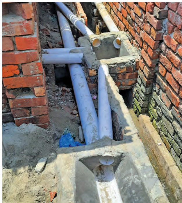
Photo 8: Underground pipe-network system
