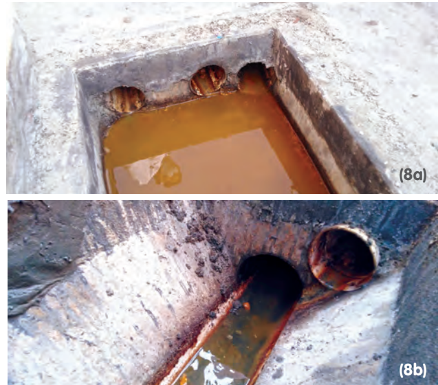
Photo 10: Sub-inspection pit (8a) and main inspection pit (8b) of the sludge collection network
